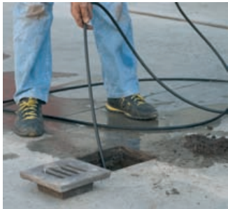
Example of the unclogging water jetter pipe in action. Thanks to the front and rear jets on the nozzle, the pipe moves along the drain.
