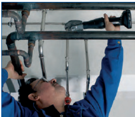
iPress MINI To work in reduced spaces
