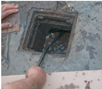
Example of the unclogging water jetter pipe in action. Thanks to the front and rear jets on the nozzle, the pipe moves along the drain.
